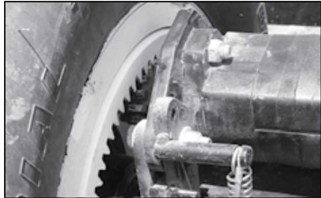
Fig 89 - Bin fill conveyor drive gears
